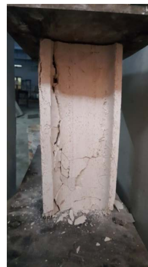
Fig.3 Failure pattern of GFRG panel
